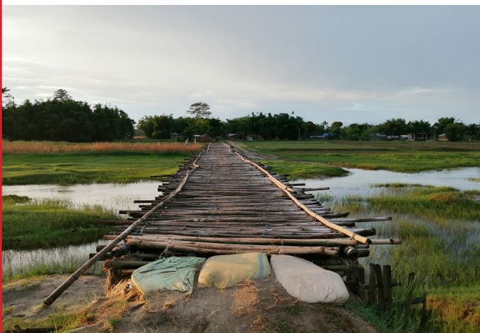
Temporary bamboo bridge used to reach school
